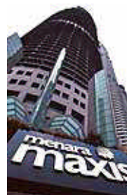
M74- MAXIS BUILDING
