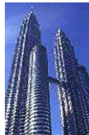
M73- PETRONAS TOWERS
