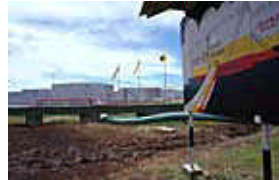
B27- OIL PLANT
