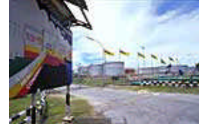
B28- OIL PLANT
